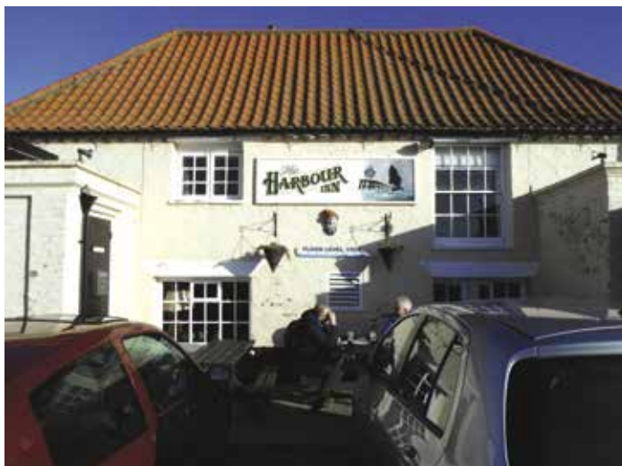
The 1953 storm surge level on The Harbour Inn, Southwold at 3.50 m above sea level. In 2013, the level on the nearby Coastguard Cottages only reached 2,76m.
