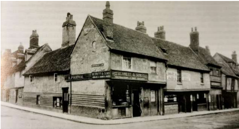
The corner of Magdalene Street and Chesterton Lane before demolition in 1911–12
